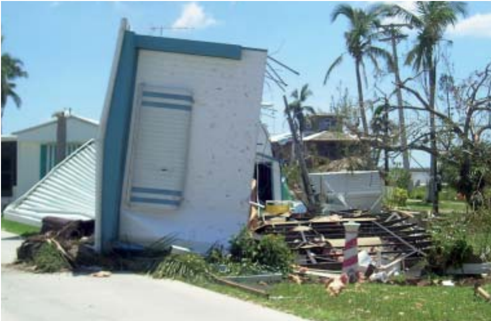
In 2004, Hurricane Charley sped over Cuba, Jamaica, the Caymans, and the US South with wind speeds of up to 240 km/h. Mobile homes like this one in Bokeelia, Florida, put up very little resistance.
