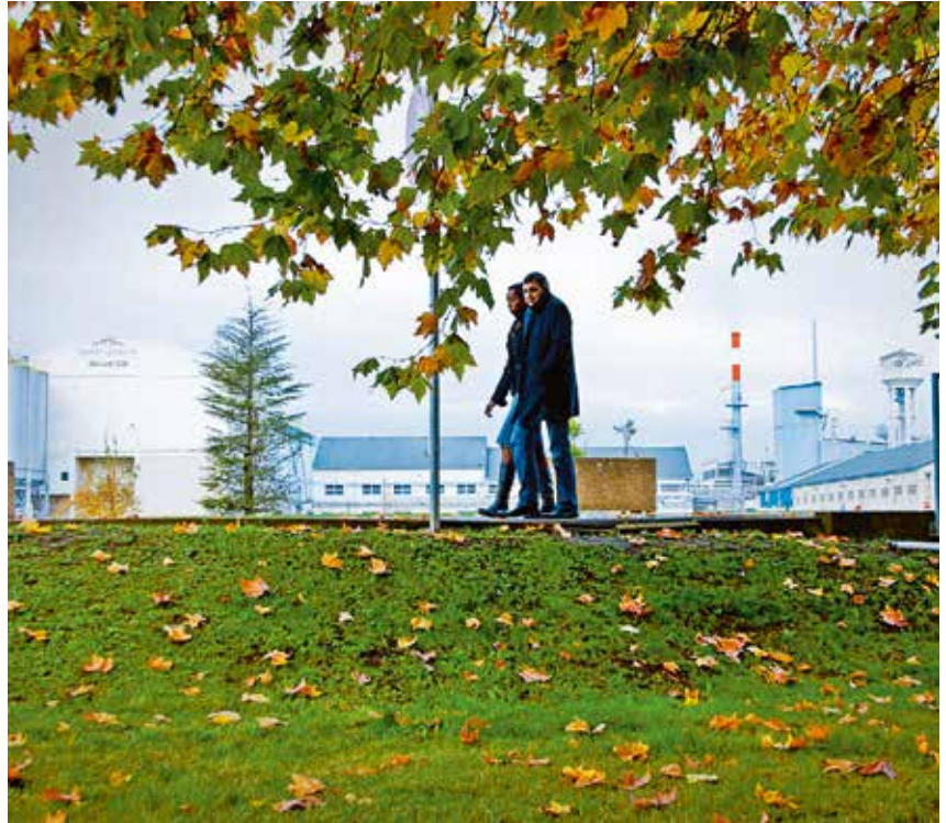
Rantigny insulation research center (France)
