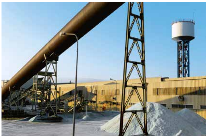
Cullet storage at the Eurofloat site (France)
