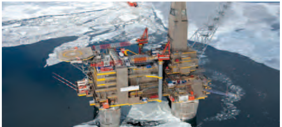
↑ Sakhalin II's Lunskeye-A platform is built to withstand huge pressures from ice floes.
