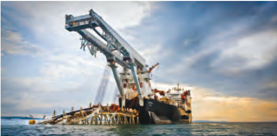
↑ Laying the offshore pipeline for the Corrib gas project, June 2009.
