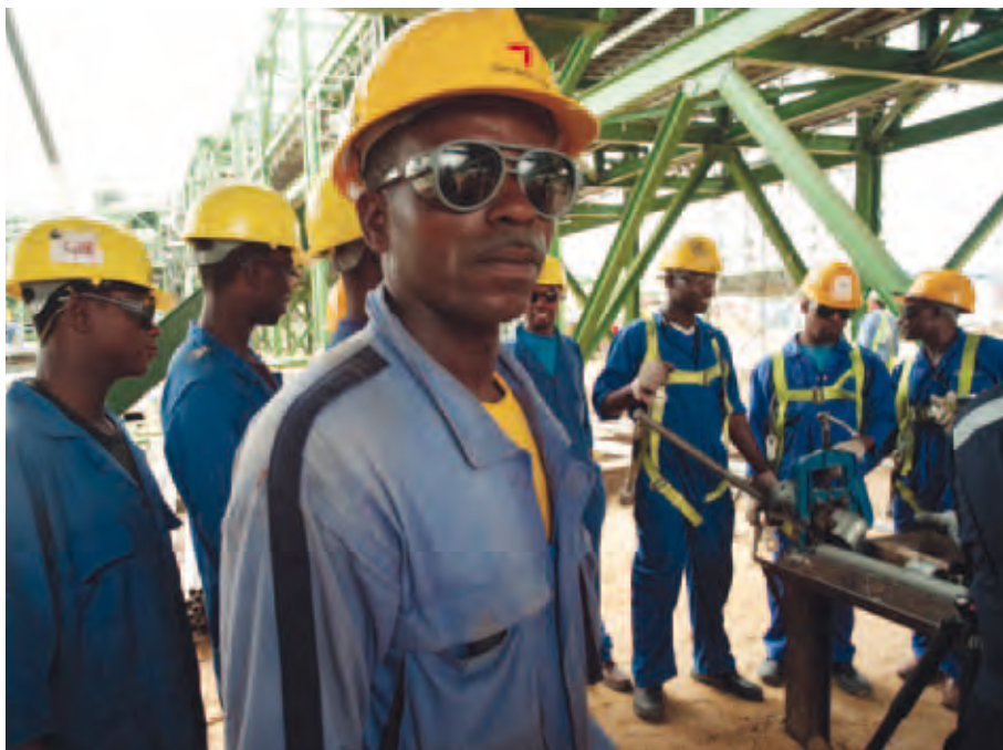
↑ Workers at the Gbaran-Ubie construction site.
