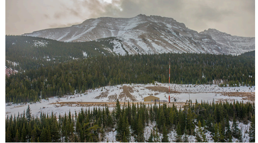
In Canada, we installed two radio towers at our Waterton shales project, which involved addressing several environmental sensitivities.
