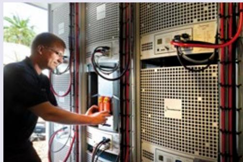
Our Platinum business has partnered in a fuel cell mini-grid rural electrification field trial in a local community near the town of Kroonstad in South Africa's Free State Province. The prototype product is fuelled with methanol and was developed for off-grid residential use, as a provider of electricity to remote communities.
