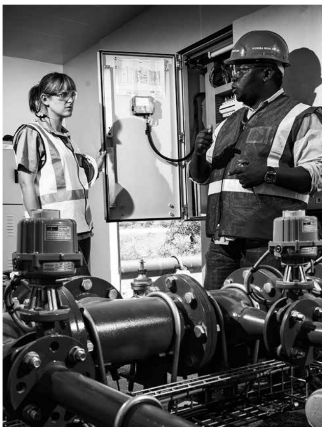
At Kumba Iron Ore's Kolomela mine, environmental technician, Islay-Jane Sparks, and project engineer, Percy Nxumalo, check the pumping station where water from the mine is fed into an adjacent aquifer.
