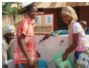
A mini water works completed this year at Iju, Nigeria, provides water for 100,000 people from 21 fetching stations
