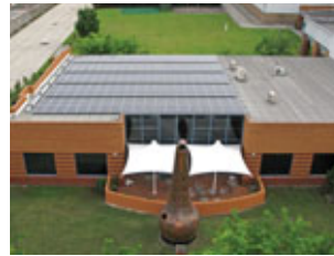
Solar panels at Huntingwood, Australia provide all of the electricity used by the site's office
