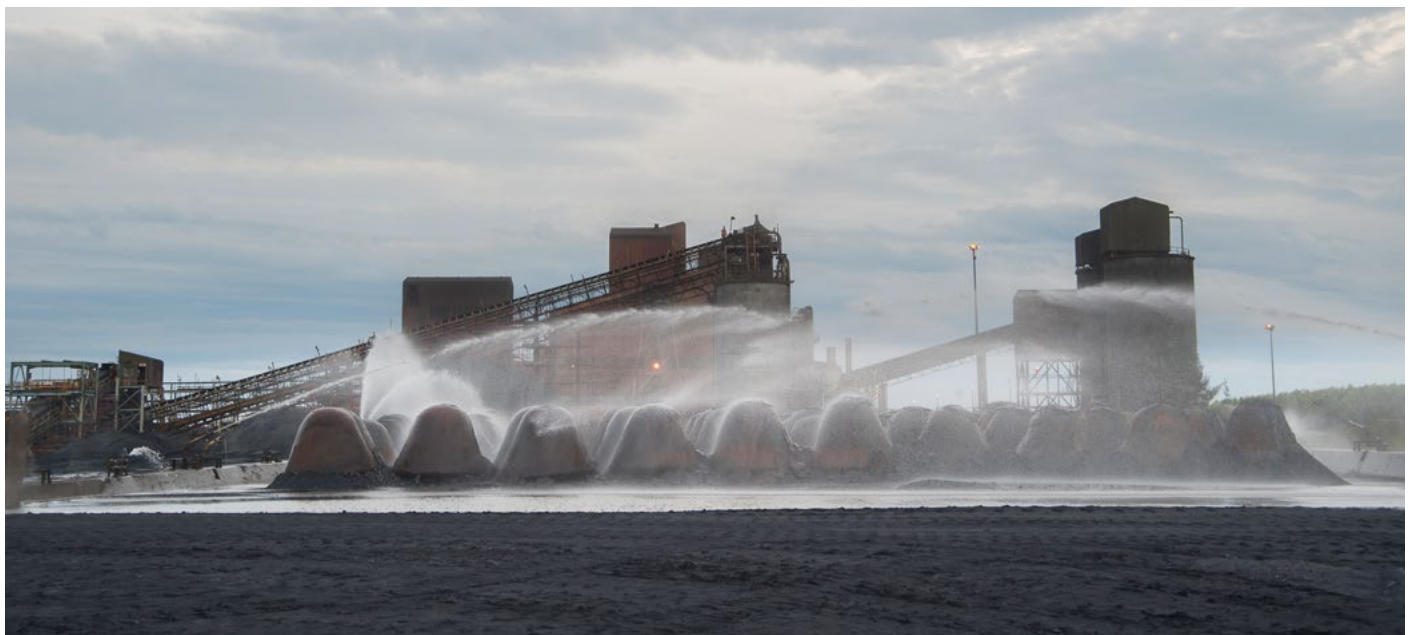
Image: Water sprinklers are used to cool down slag, Richards Bay Minerals, South Africa
