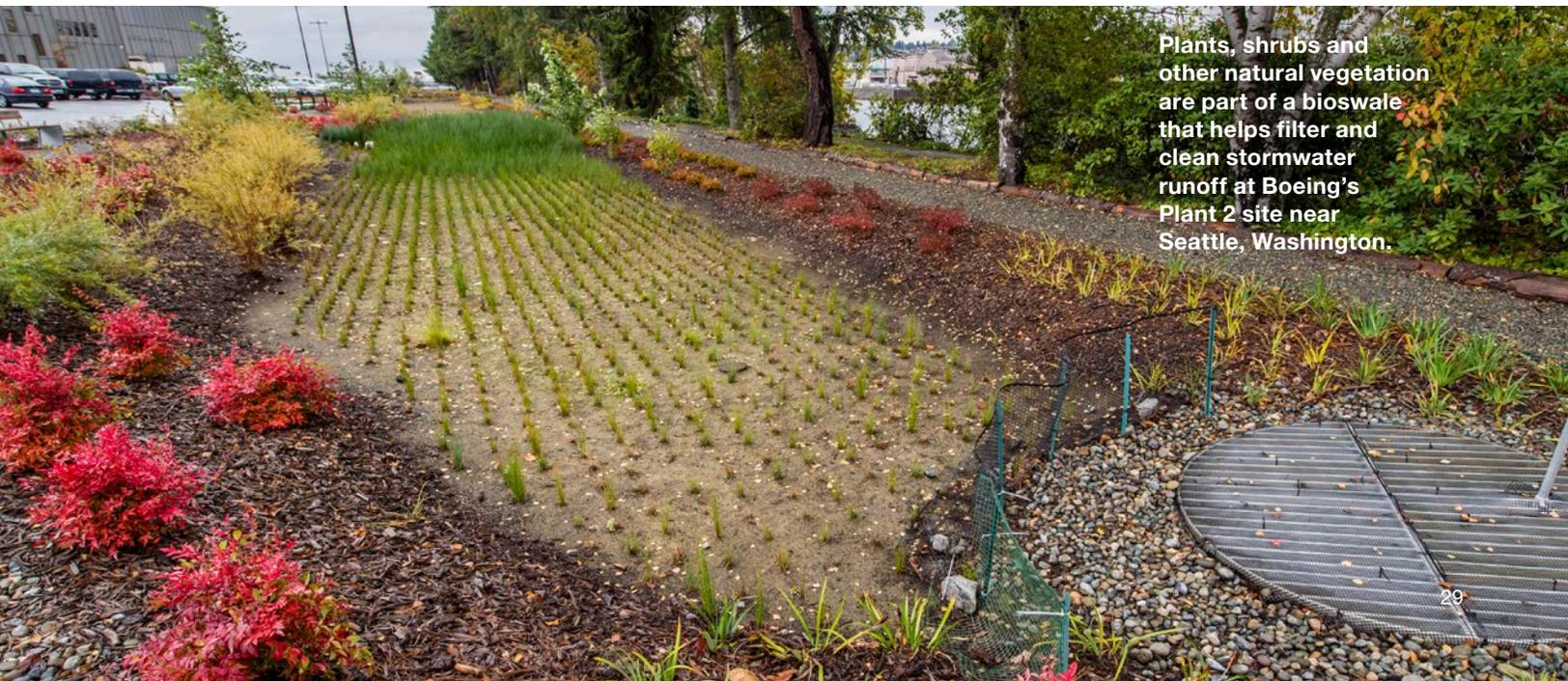
Plants, shrubs and other natural vegetation are part of a bioswale that helps filter and clean stormwater runoff at Boeing's Plant 2 site near Seattle, Washington.
