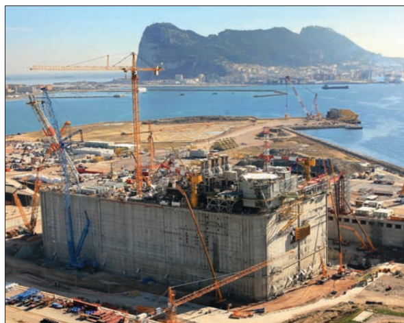
The Adriatic LNG terminal will be the world's first fixed offshore storage and regasification terminal. It is under construction in Spain and will be transported to Italy's Adriatic coast in 2008.
