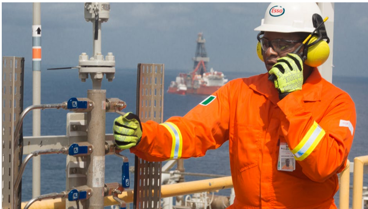
Kanu Okechukwu, a production operator for Esso Exploration and Production Nigeria Limited, opens a manual valve to supply compressed air to equipment at the Erha North phase two project in Nigeria.
