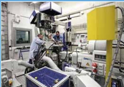
Two Powertrain Engineering Development Centers are regenerating excess energy back into the grid to help power their facilities.
