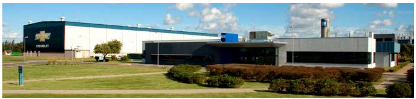
A combination of global principles and local policies guide GM's environmental stewardship at facilities such as the Rosario Auto Complex in Argentina, the first GM plant in the Americas to obtain ISO 50001 Energy Management certification.
