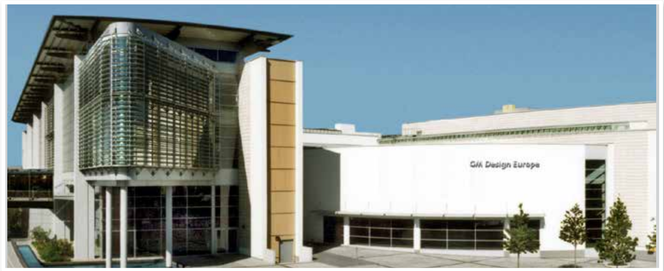
Our Environmental Management System drives continuous performance improvement while satisfying legal requirements, and corporate and site-specific objectives and targets.
