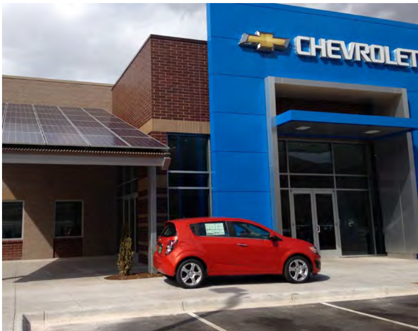
Mountain Chevrolet in Glenwood Springs, Colorado, earned Green Dealer certification, thanks in part to a 40-kilowatt solar array that supplies power to the dealership.
