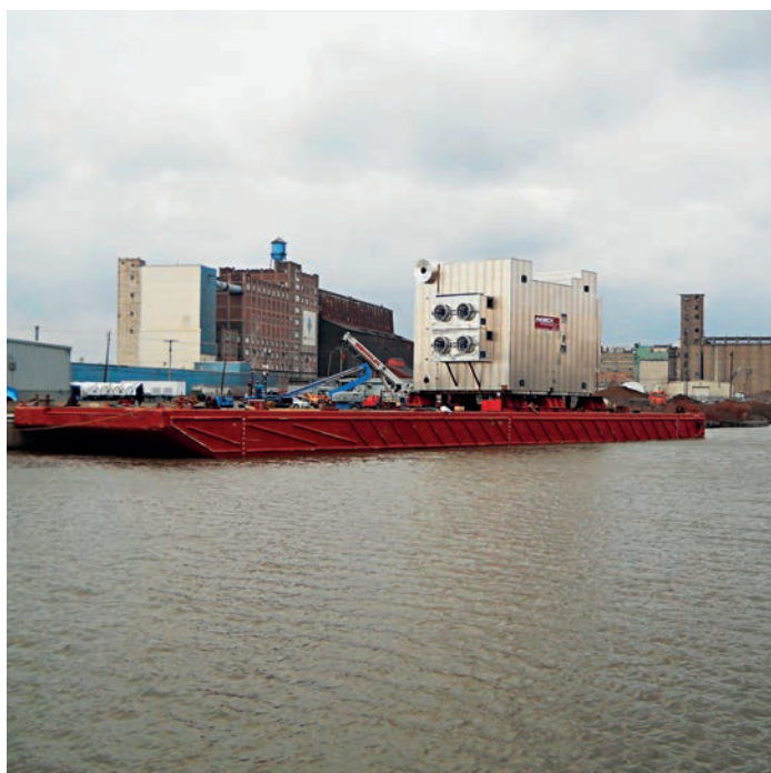
The 504 Boiler, on a barge in Buffalo, New York set on its way to a new home at Indiana Harbor in East Chicago, Indiana to help drive greater energy efficiency.
