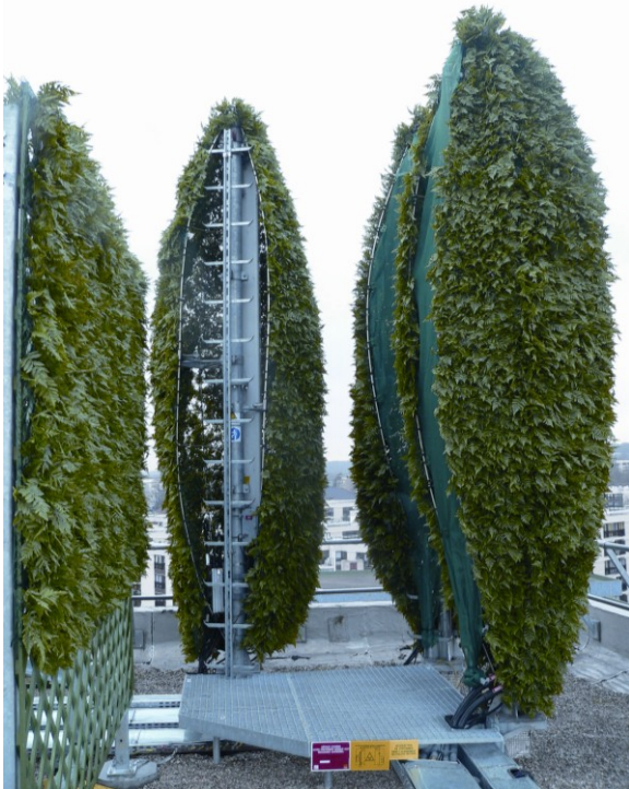
Example of landscape integration of antennas on a town hall roof in the municipality of Le Chesnay (Yvelines, France).
