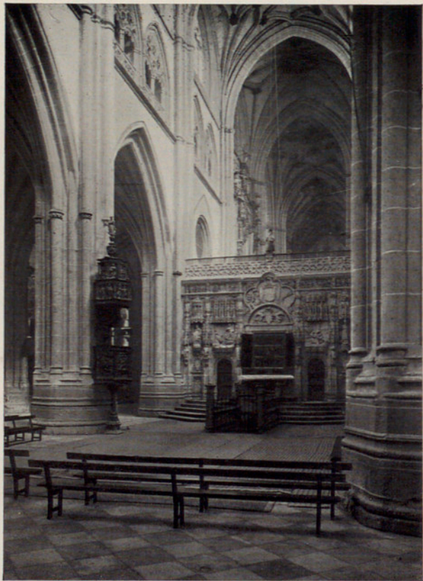
CATEDRAL. NAVE PRINCIPAL
