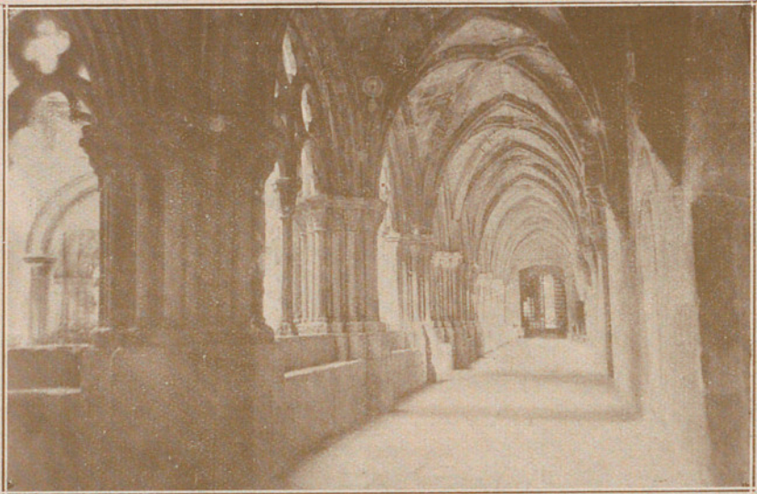
Claustro mayor : Nave del Refectorio
