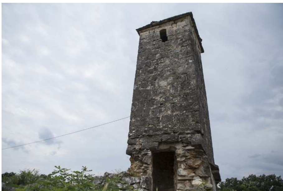
Fig. 1. Minaret in Bileća, 16th century. Source: https://vakuf.ba/bs
