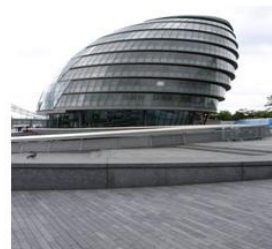
City Hall, London (steel structure)
