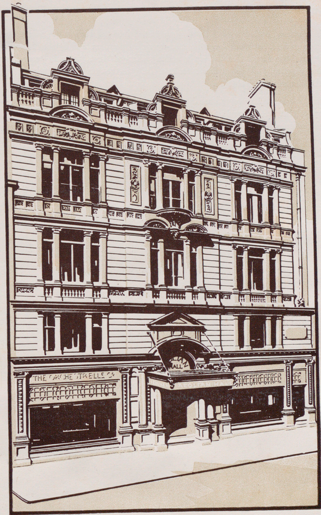
EXTERIOR OF ÆOLIAN HALL
