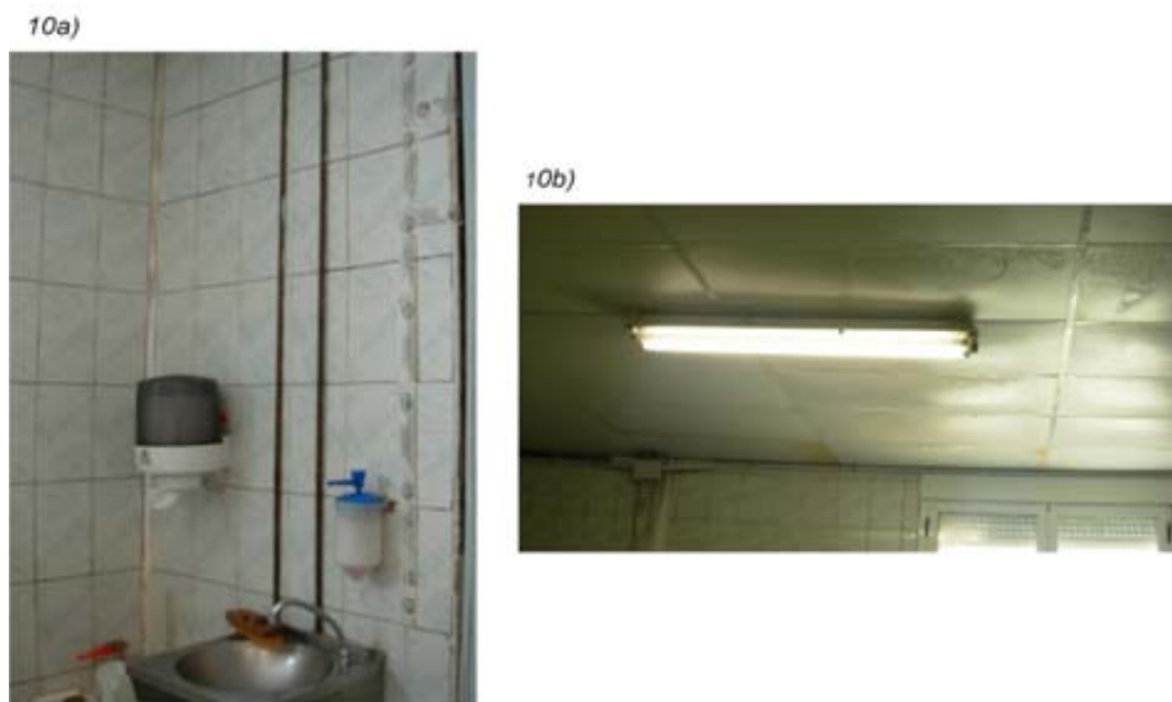
Figure 10. ECF work room
