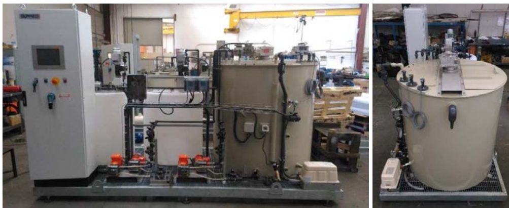
Figure 3.14: Lateral view of the pilot reactor (left) and front view of the pilot reactor (right).
