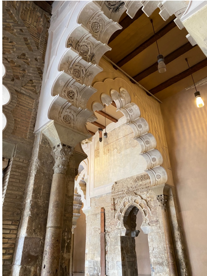
Figure 76. An angle of the north portico showing various original materials of the Taifa palace
