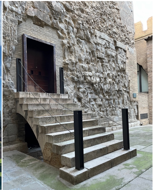
Figure 6. The current entrance to the Troubadour Tower
