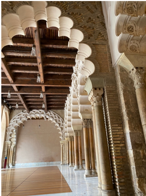
Figure 69. View of the arches of the north side
