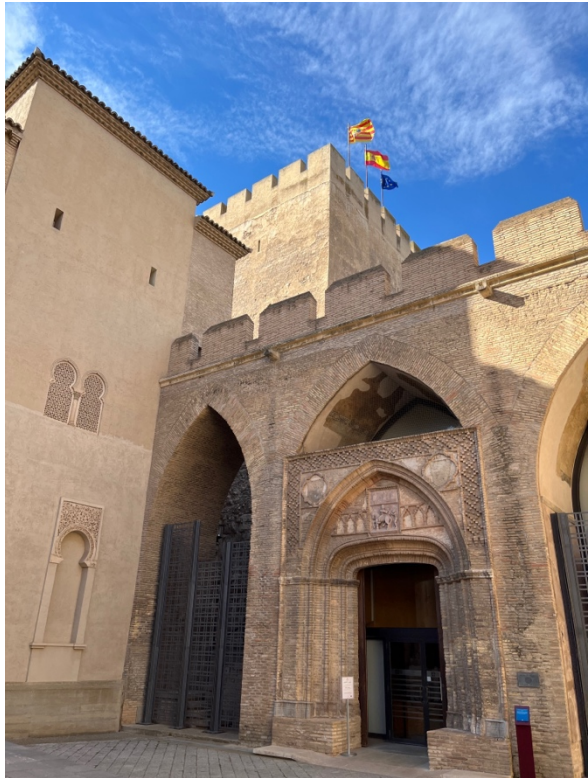
Figure 47. Saint Martin's courtyard, Showing Saint Martin Chapel, and the Troubadour Tower, the Aljafería
