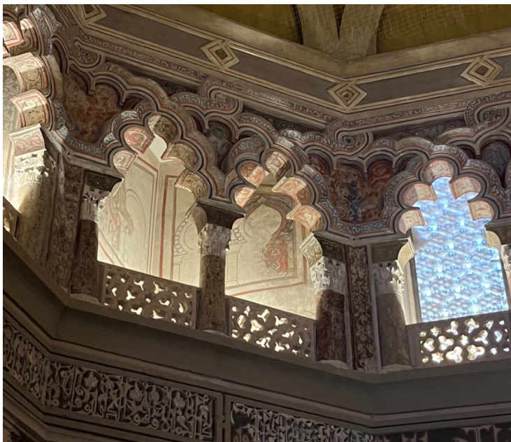
Figure 25. Details showing remains of the polychromed colors of the arches, the mosque of the Aljafería
