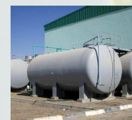
Figure 10. CO 2 2- storage tank
