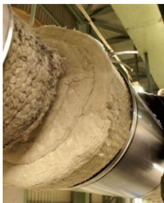
**Figura 4.2.** Lana de roca *TECH Wired Mat MT 6.1*.
