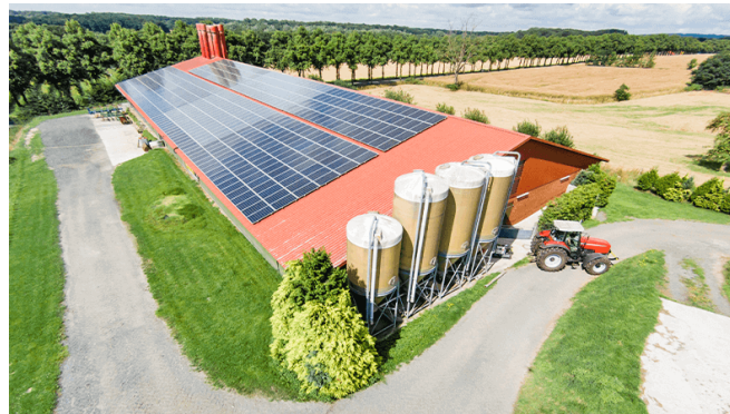
Figure 51: Solar panels Source: Tierra
