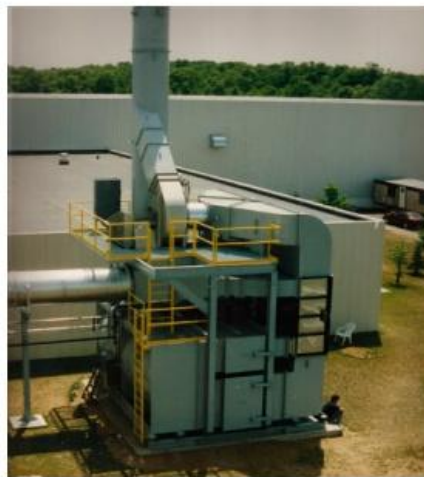
25,000 SCFM Catalytic Oxidizer with preheat exchanger (8 Weeks Deliv.)
