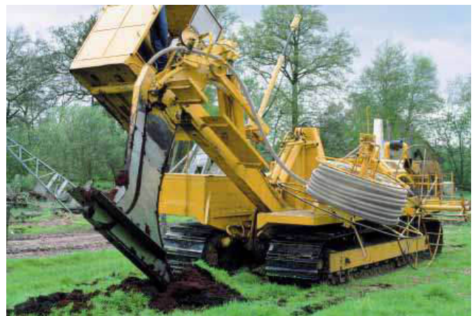
Fig. 28 Ploughing-in technique
