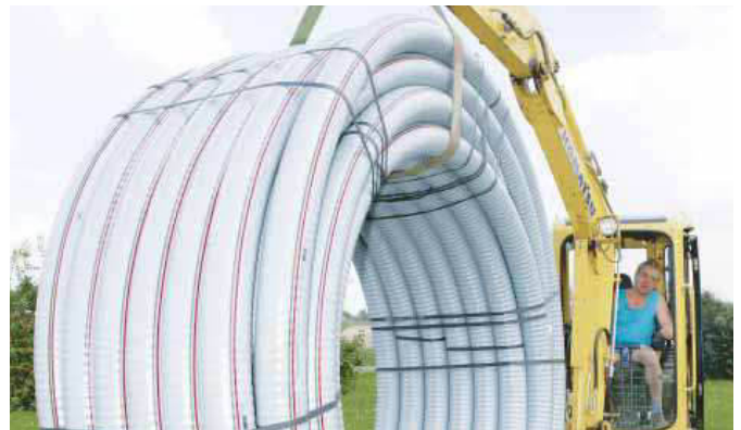
Fig. 39 Lifting with a digger
