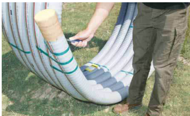
Fig. 42 Cutting the coil straps
