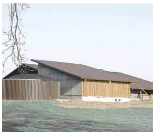
Biogas facility in Loorenhof, Switzerland
