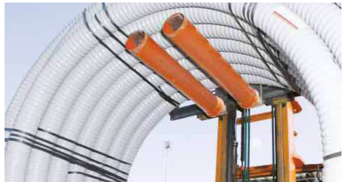
Fig. 40 Lifting with a forklift
