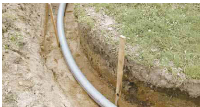
Fig. 45 Laying a bend area
