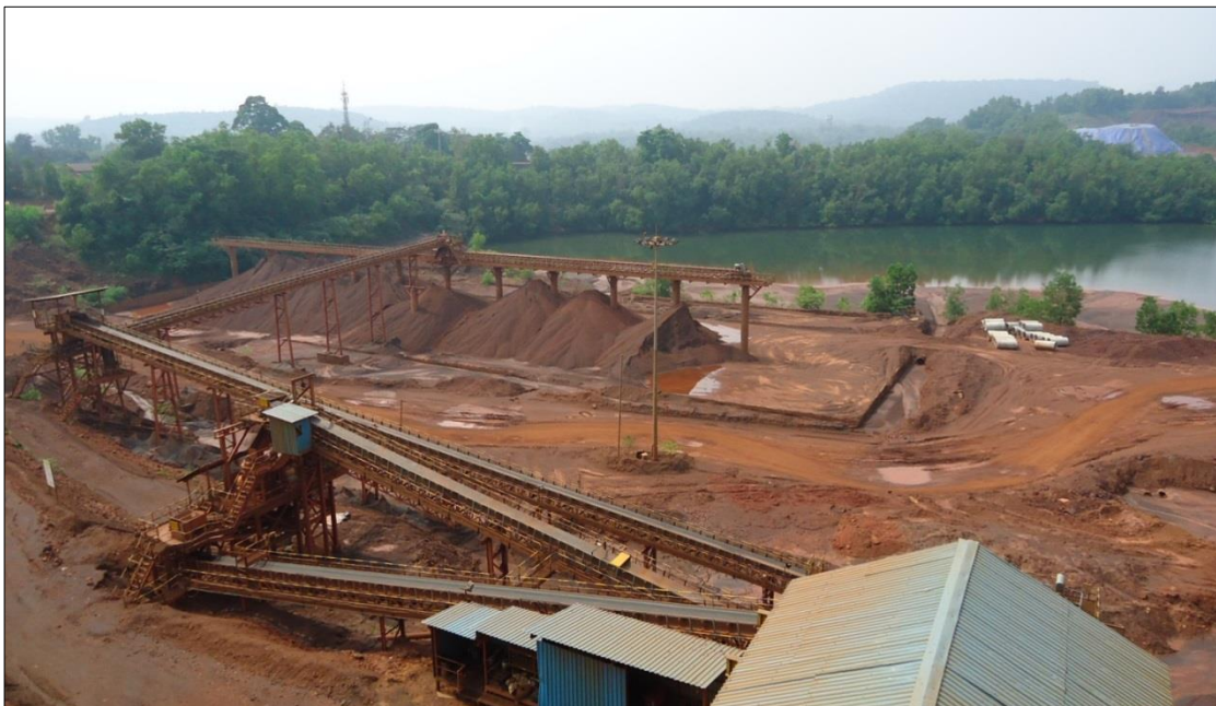
Figure 2: Crashing plant of Iron ore
