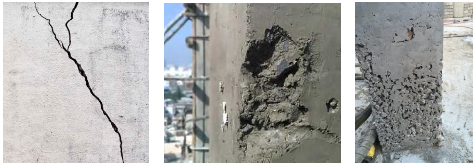
Figure 2: Examples of low-quality concrete.
