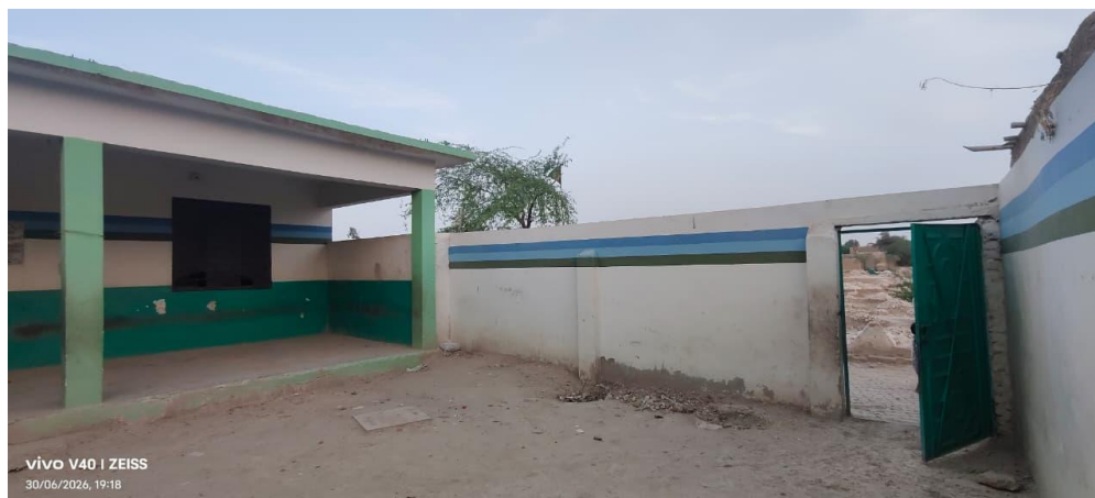
(a) School with boundary wall
