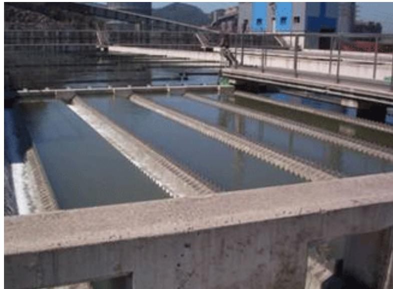
Wastewater Treatment Plant biological reactors where a complex population of microorganisms is grown degrading the organic matter of the wastewater. In this work, researchers have studied a possible way to eliminate, as well as organic matter, nitrogen and phosphorus, two elements that affect nutrients richness of ecosystems.
